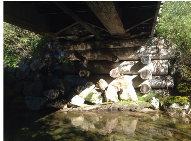
Left Bank Abutment when facing downstream
