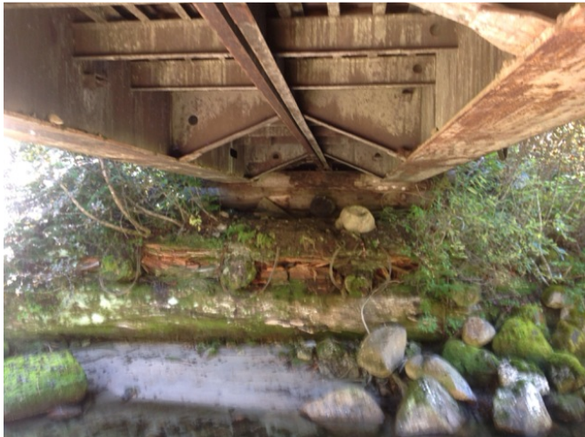
Right Bank Abutment when facing downstream
